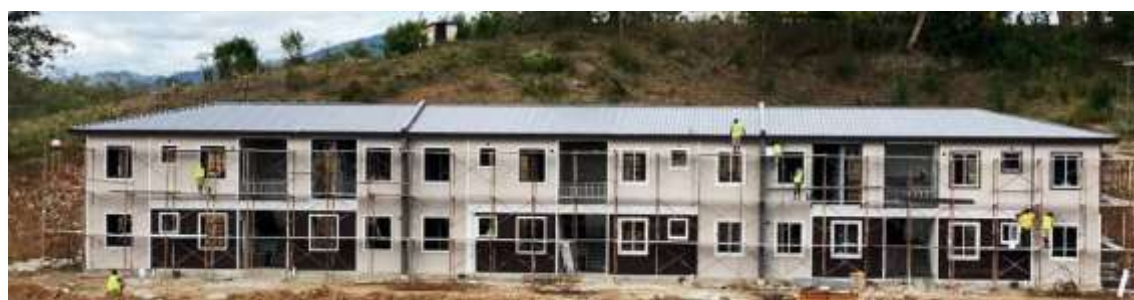
Staff housing improvement program at Tiaba, Sagalau and other Ranches in 2024 and 2025
