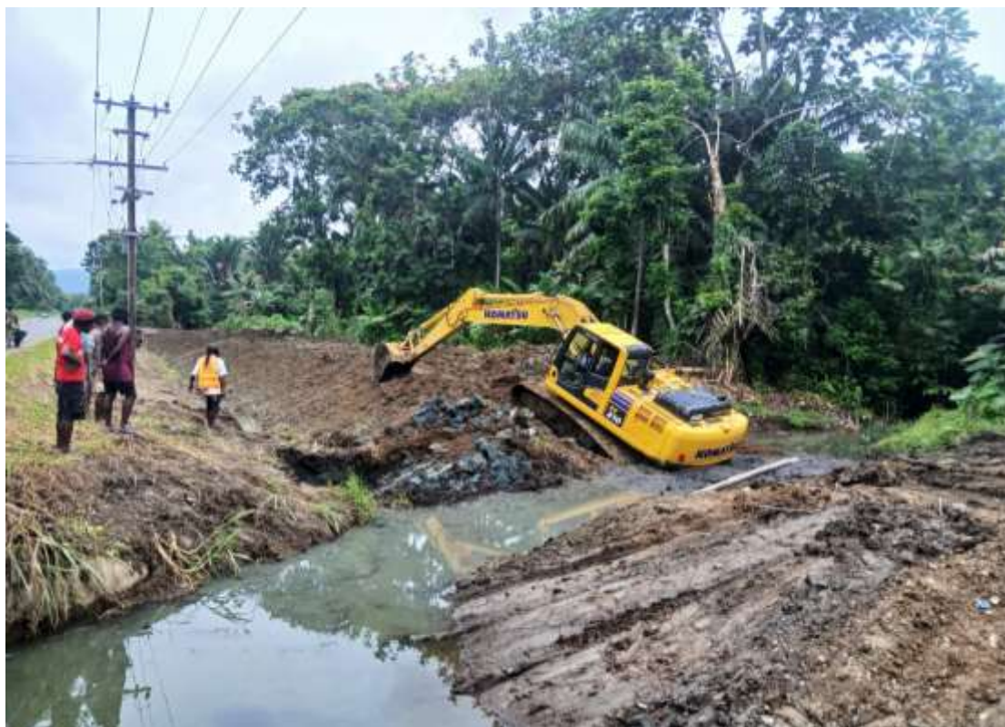
Figure 15: Excavator working to improve drainage at Wariman Station, ESP
