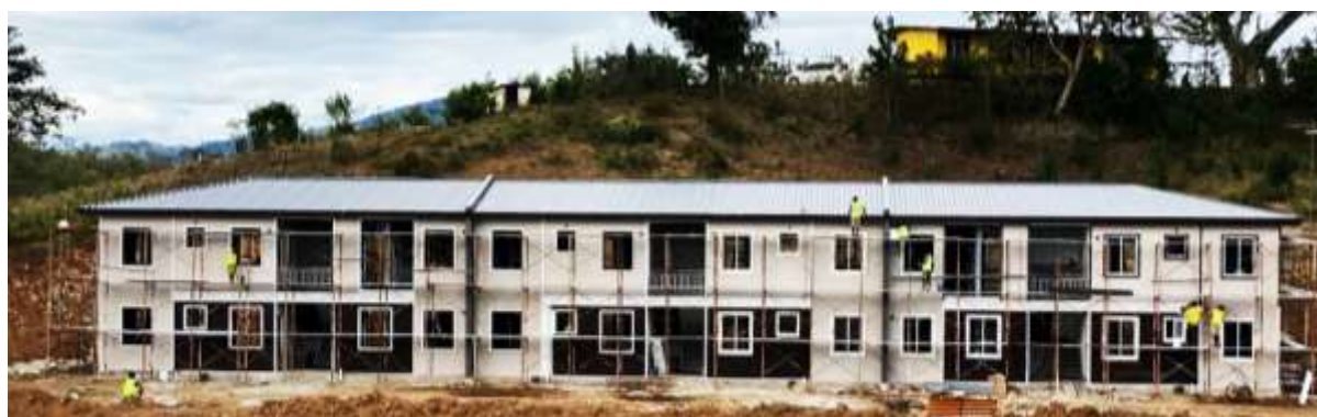
Figure 7: Staff Accommodation under construction at Tiaba, 12-mile NCD, 2025
